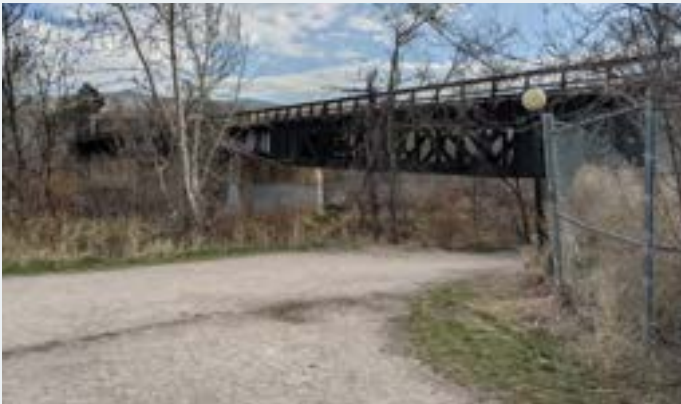
Existing Montana Rail Link Trestle
