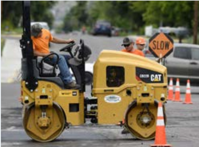
Construction work in Missoula
