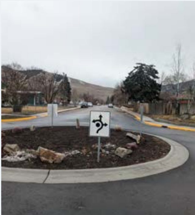
Installed neighborhood greenway elements
