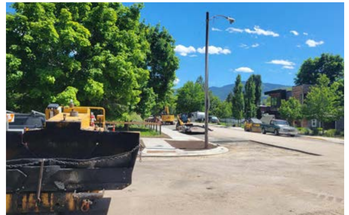
Construction of the Ivy Street/Franklin Neighborhood Greenway
