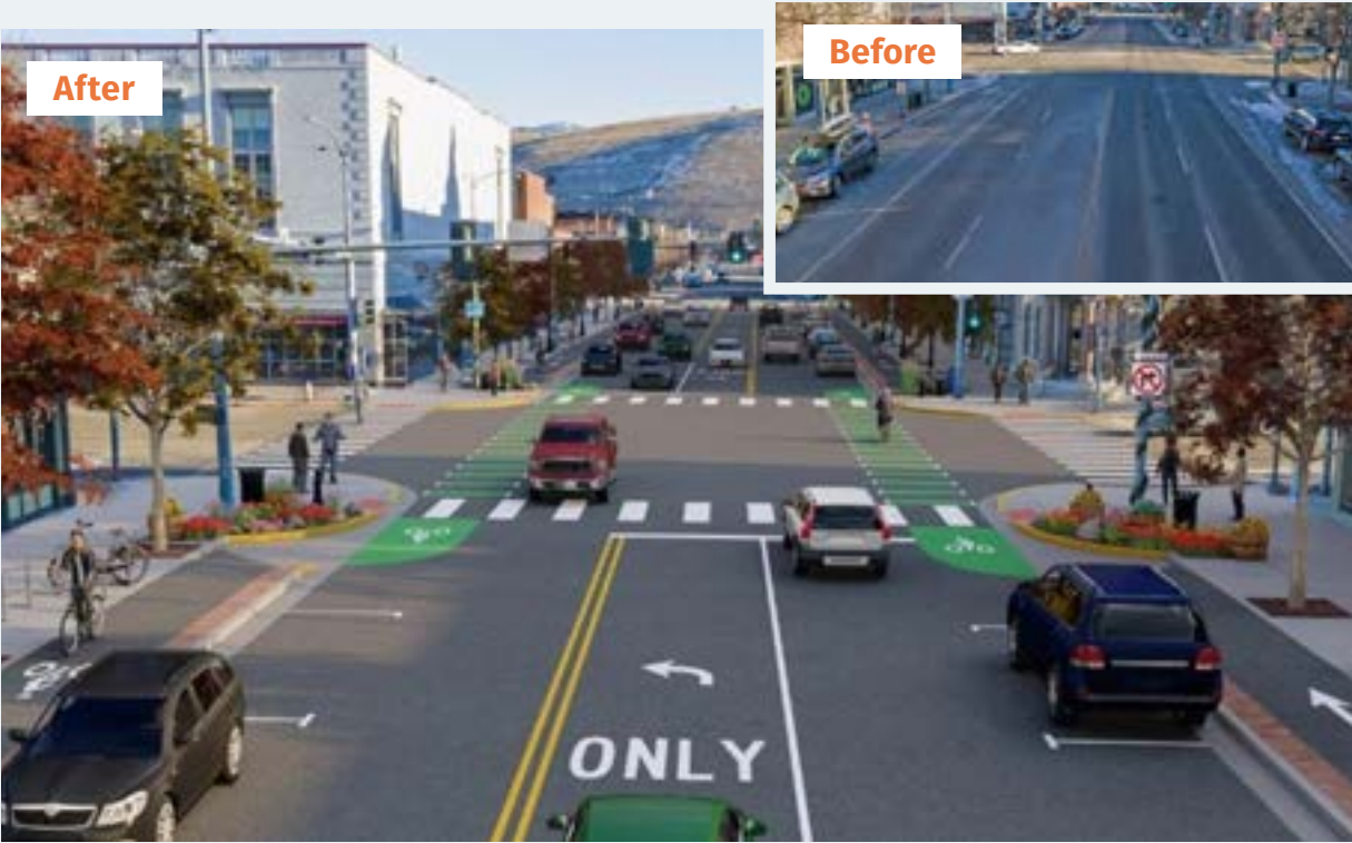
Higgins Avenue Street Improvements
