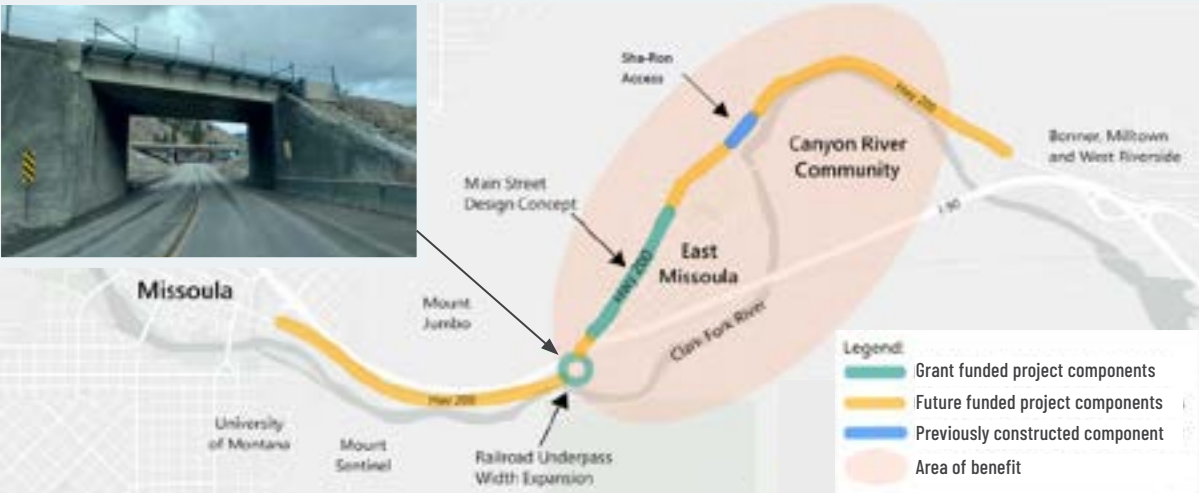
Railroad underpass location and its existing condition
